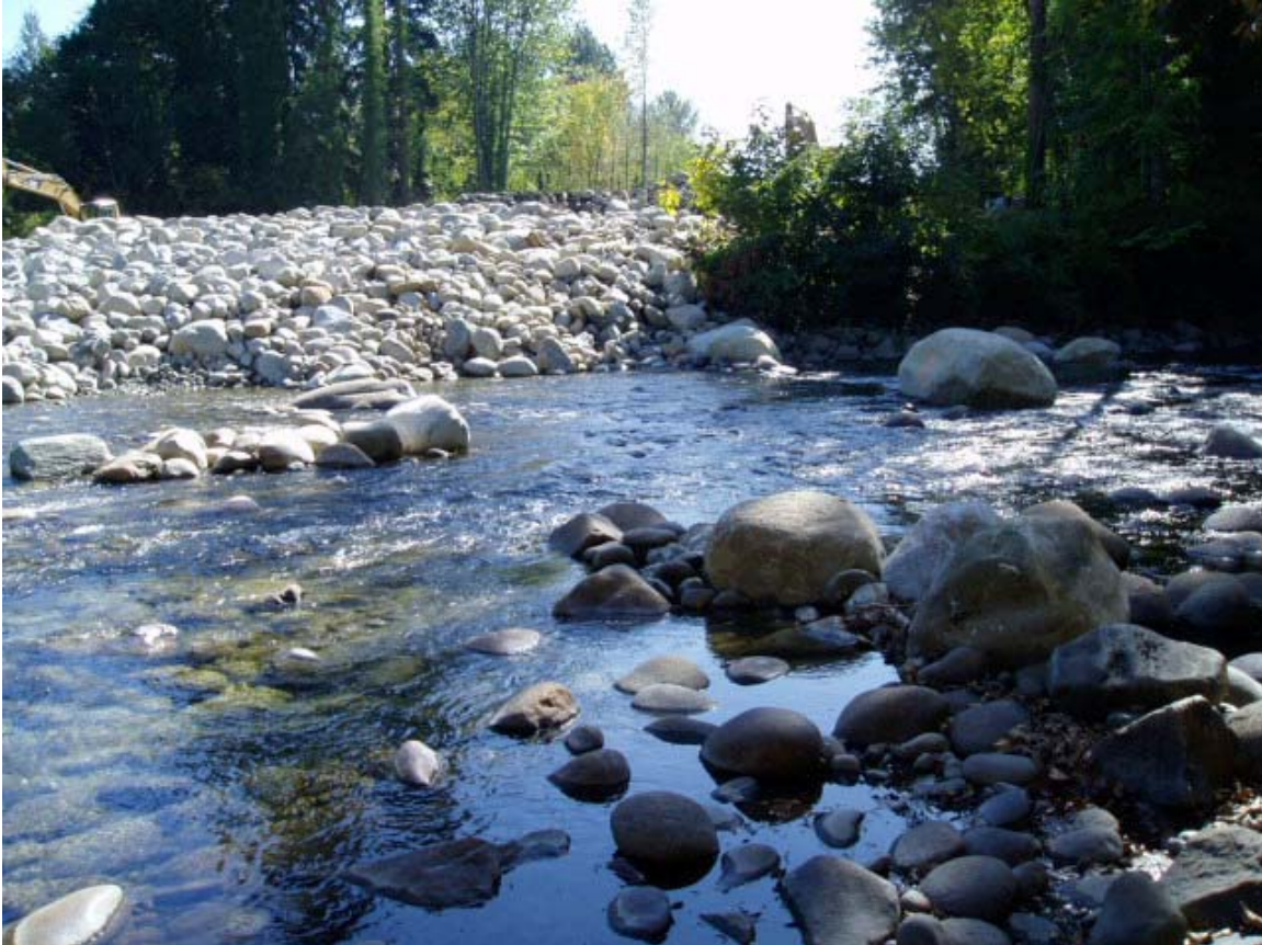
Photo 3 – Boulders installed in September 2006, downstream of water main.
